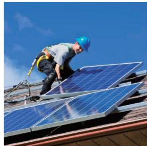
Perform load rejection testing of solar power systems
